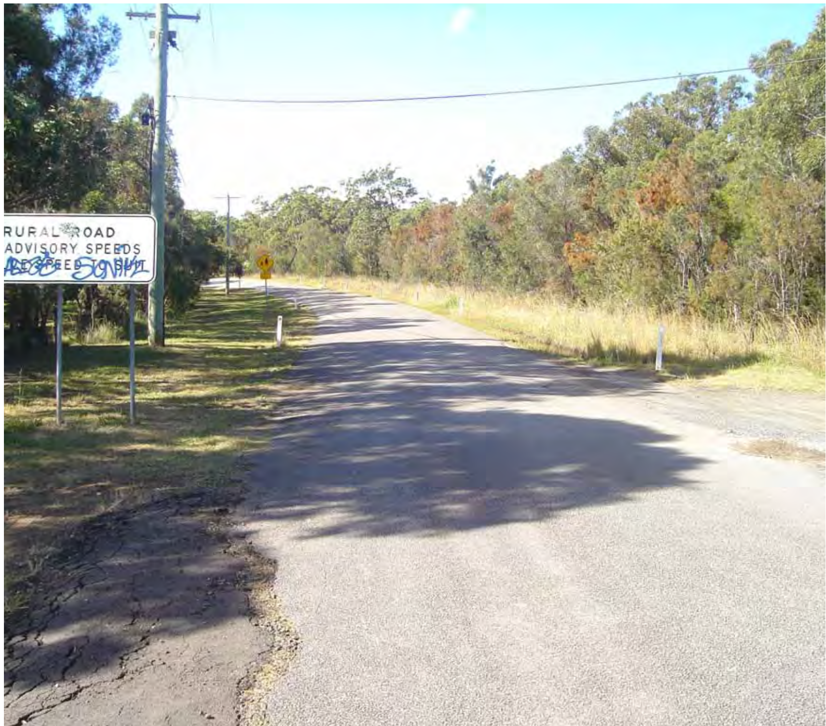
Photograph 5 – Bushells Ridge Road near F3 overpass
