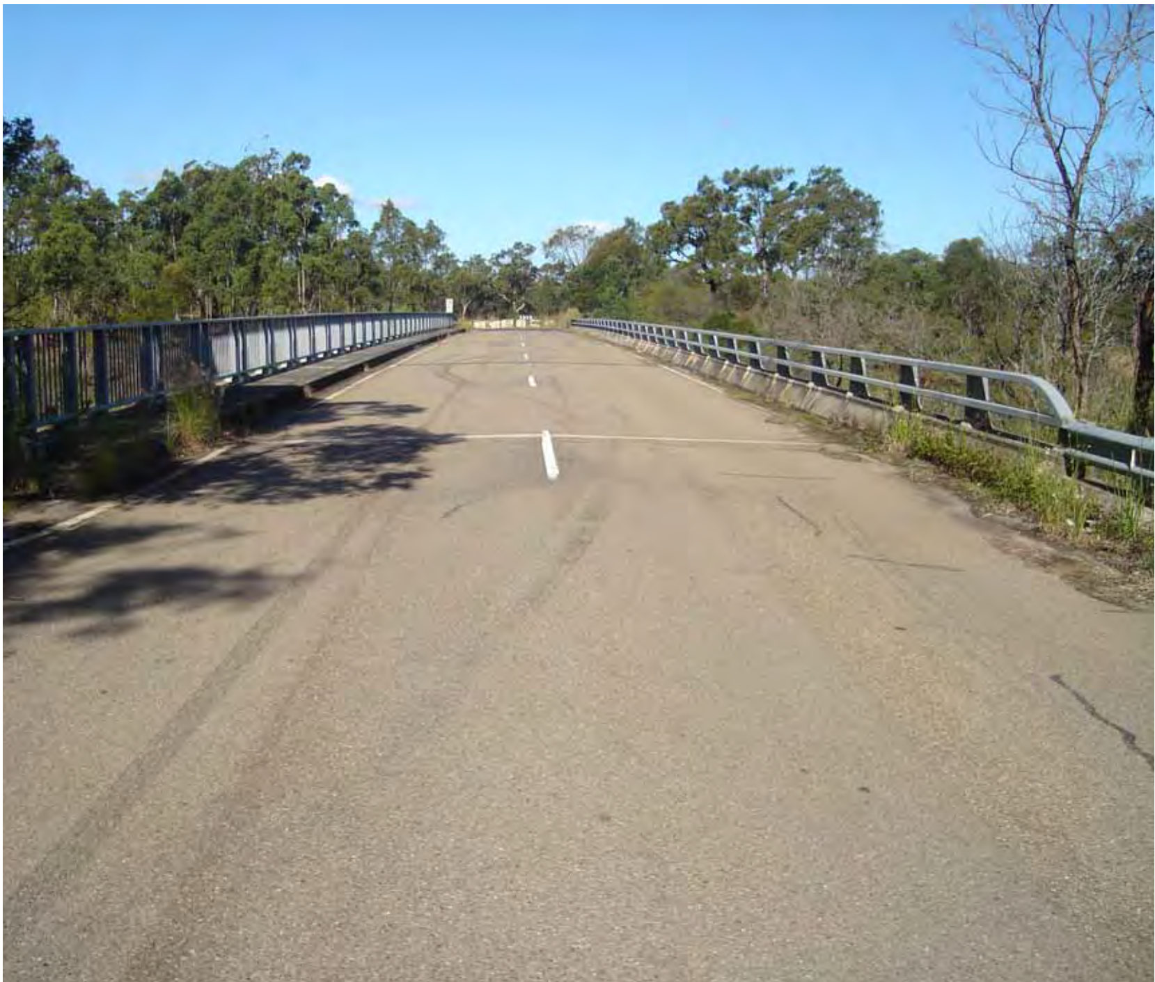
Photograph 1 – Tooheys Road overpass (Motorway link Road) near proposed Wallarah Estate
