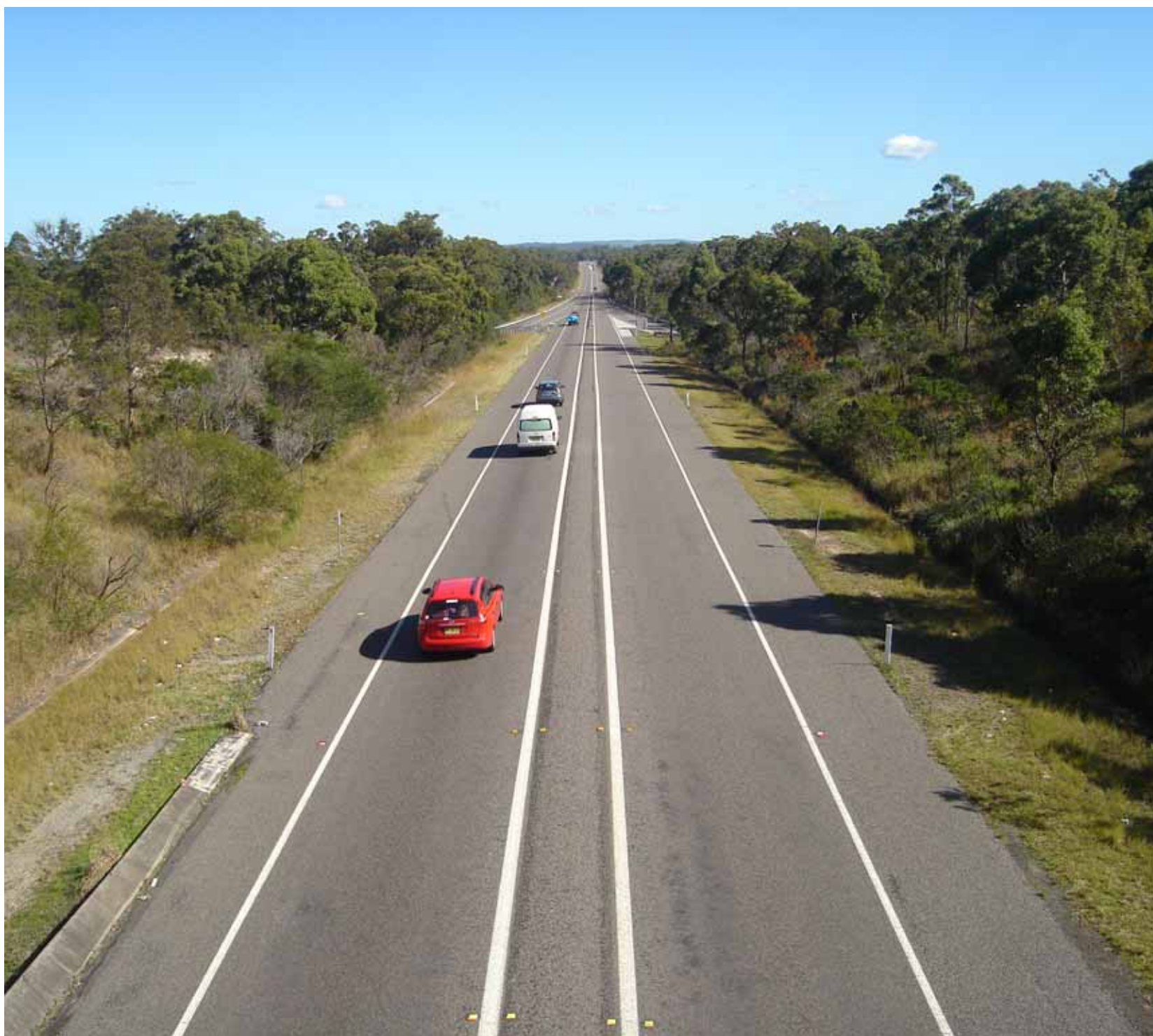
Photograph 4 – Motorway Link Road (MR 675) near Tooheys Road interchange
