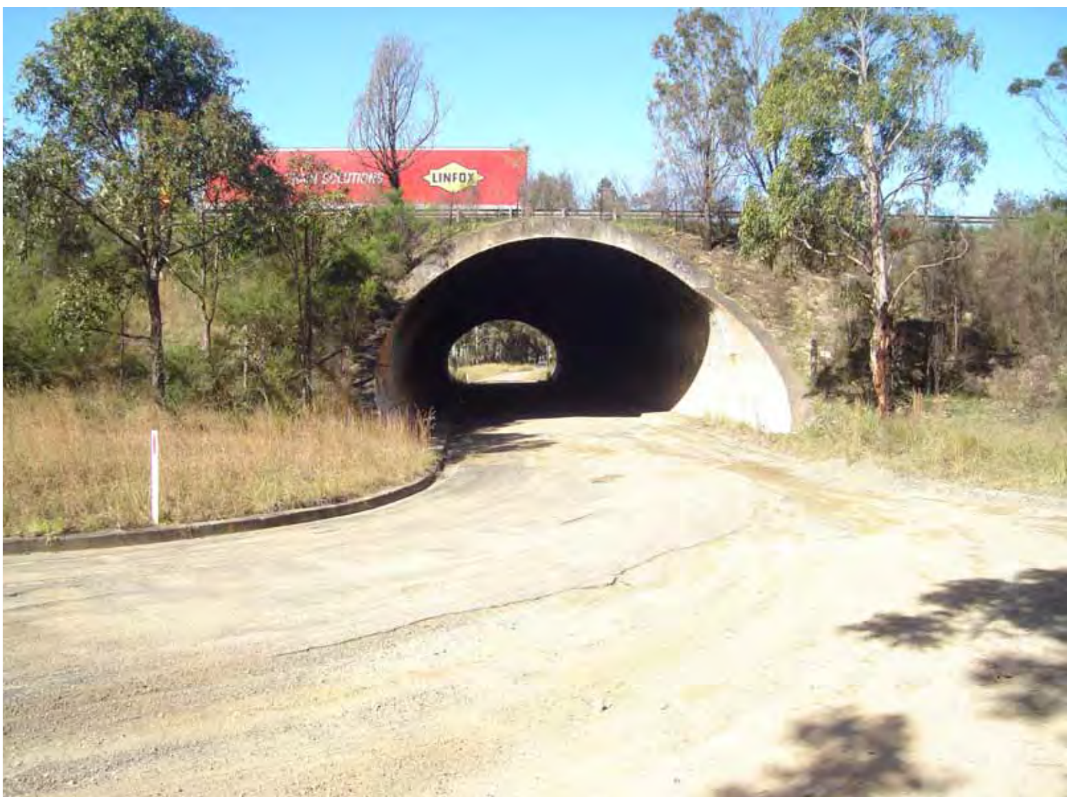
Photograph 3 – Tooheys Road underpass (F3 Freeway)
