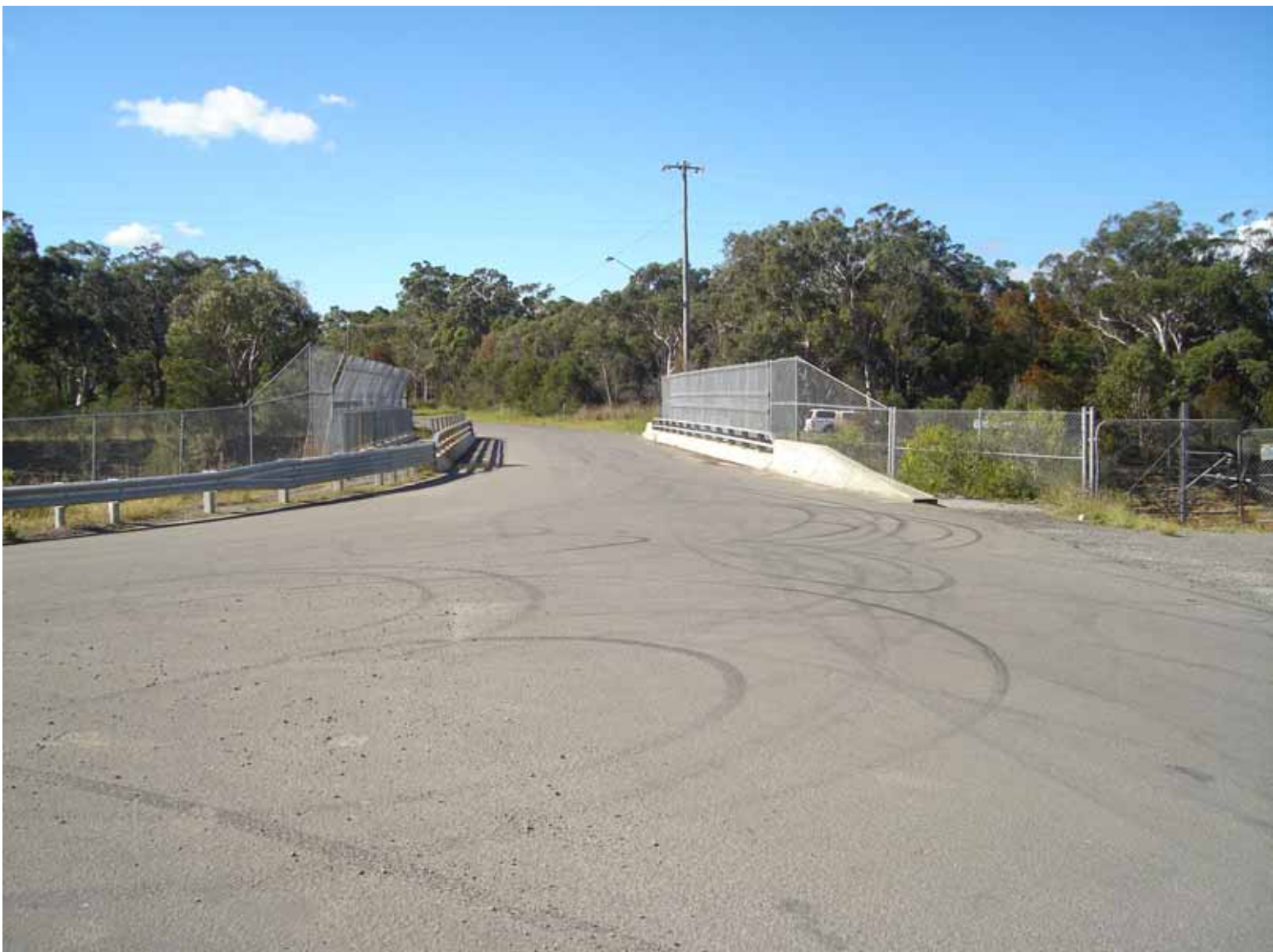
Photograph 7 – Northern Railway Line overpass – Bushells Ridge Road
