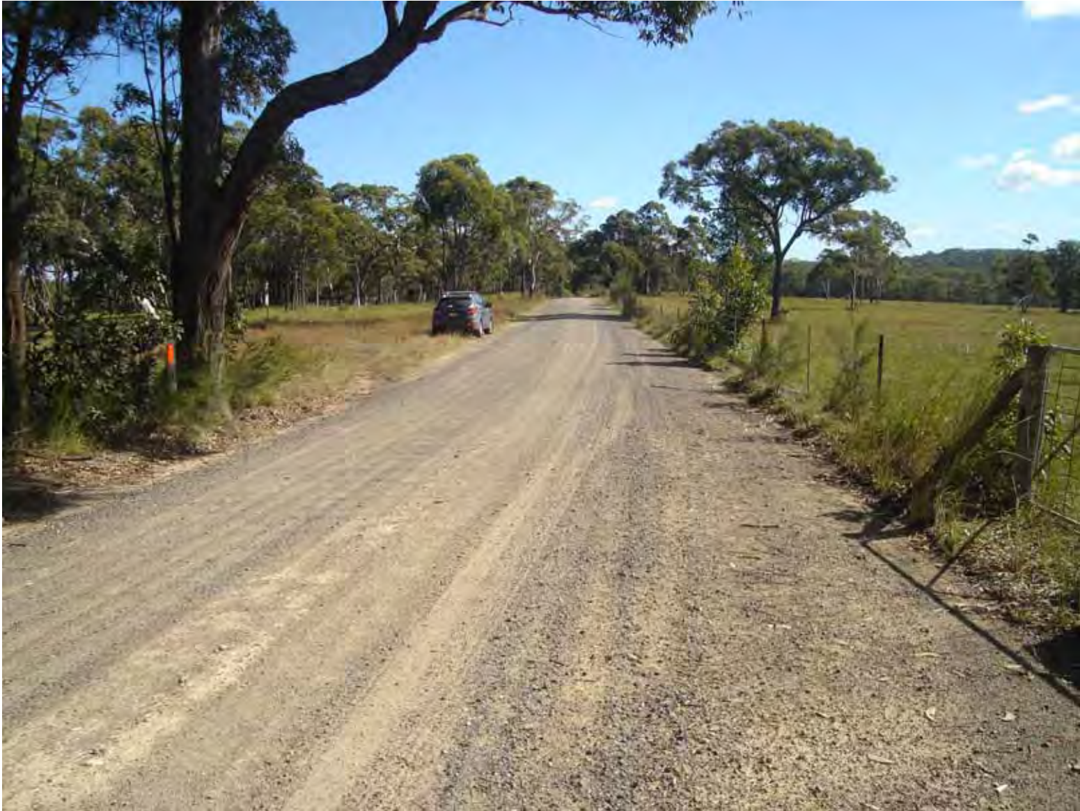
Photograph 2 – Tooheys Road west of Boral Quarry near proposed Bushells Ridge Employment Estate access.
