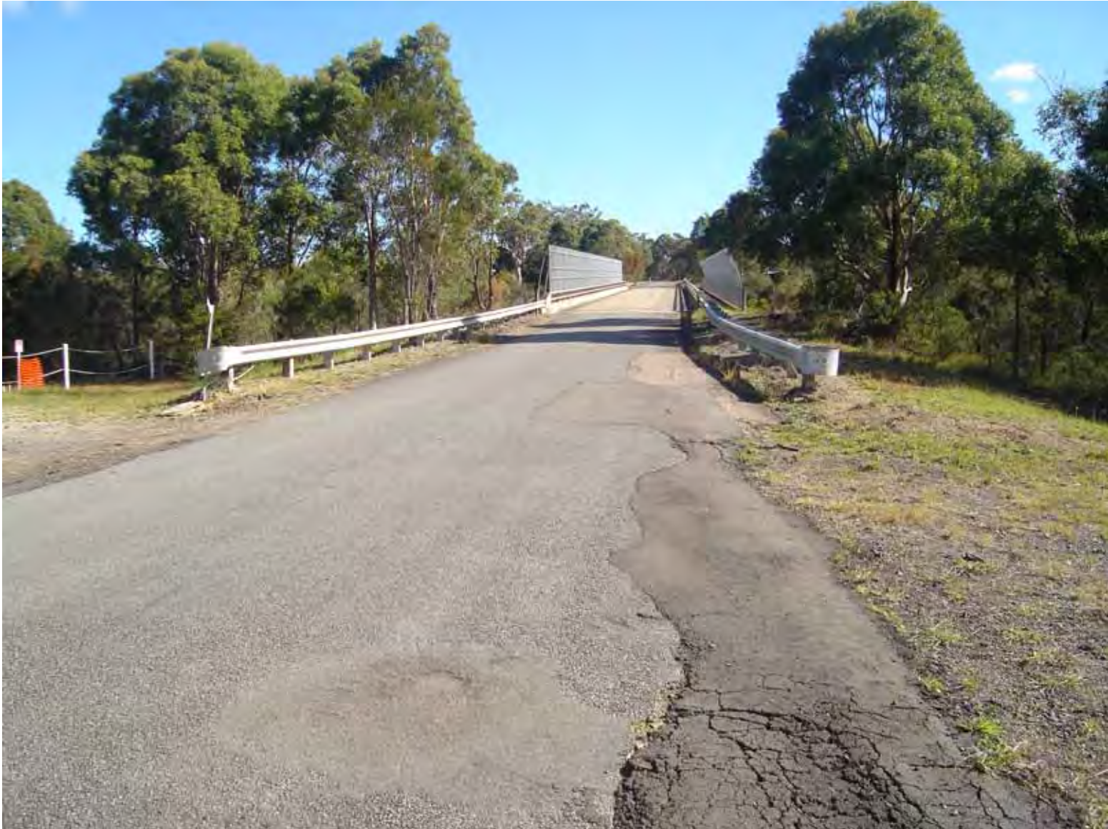
Photograph 6 – F3 overpass – Bushells Ridge Road
